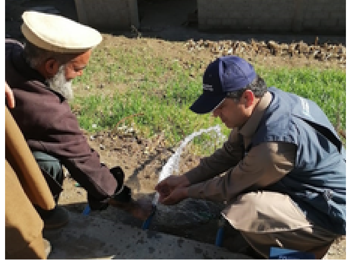
Monitoring of Water Scheme at Motatangi Shangla
