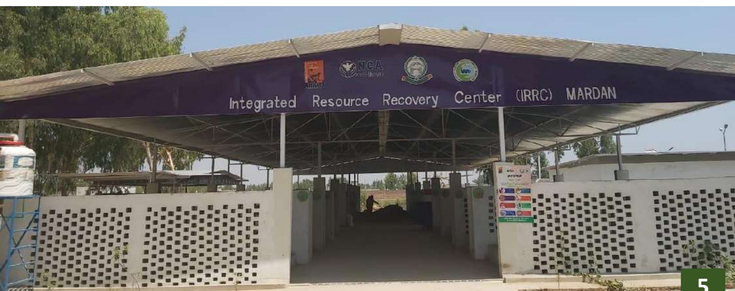
NCA handed over of Waste Management Facility to Water and Sanitation Company Mardan, KP
